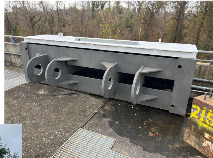
Valve Trunnion Beam
