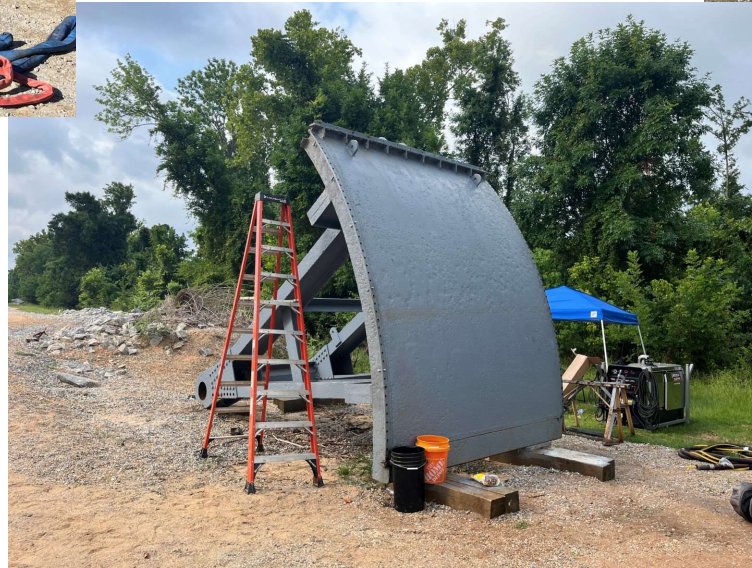
Blasted & Painted Valve
