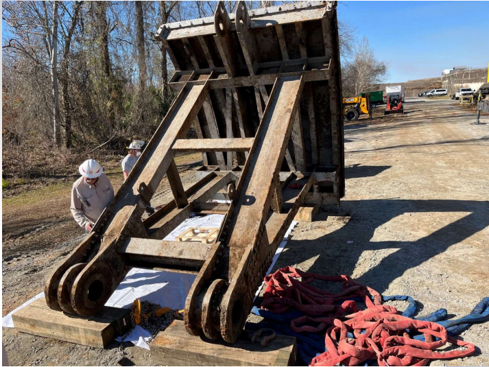
Original Valve Condition
